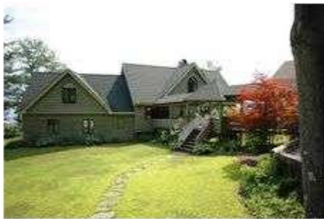
Road side view
